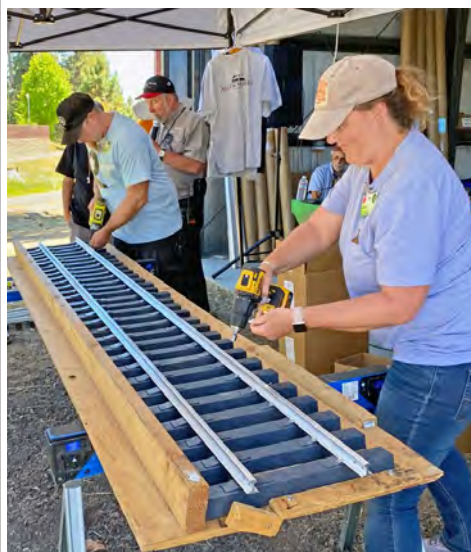
▼ Building track panels using Accu-Tie track system at the Train Mountain Triennial
